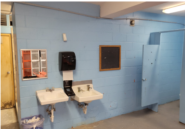
Fig. 3.4.71: Lower Level Locker Room, 2023.
