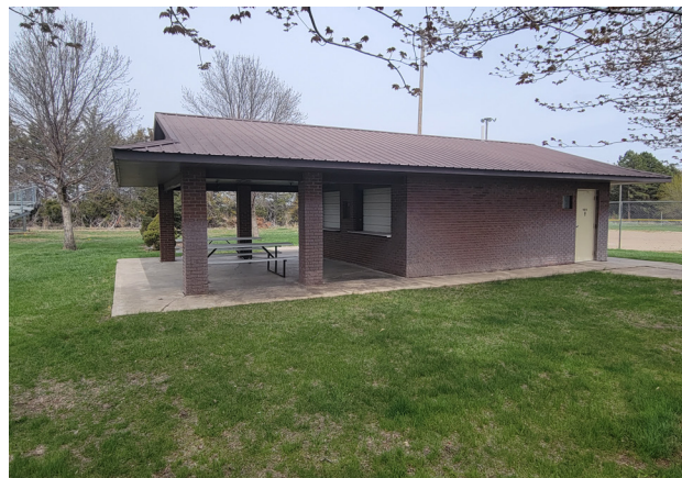
Fig. 3.4.15: Concession and Restrooms, 2023.
