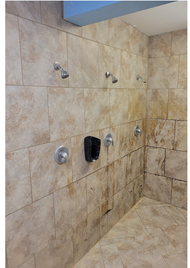
Fig. 3.4.73: Lower Level Showers, 2023.
