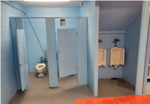
Fig. 3.4.69: Lower Level Locker Room, 2023.
