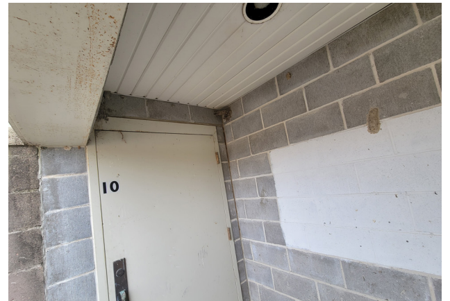
Fig. 3.4.30: Exterior Soffit and Door, 2023.
