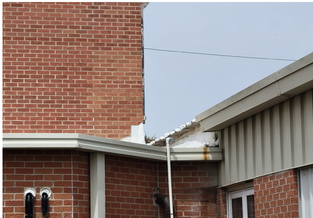
Fig. 3.4.29: Roof Spray Coating, 2023.
