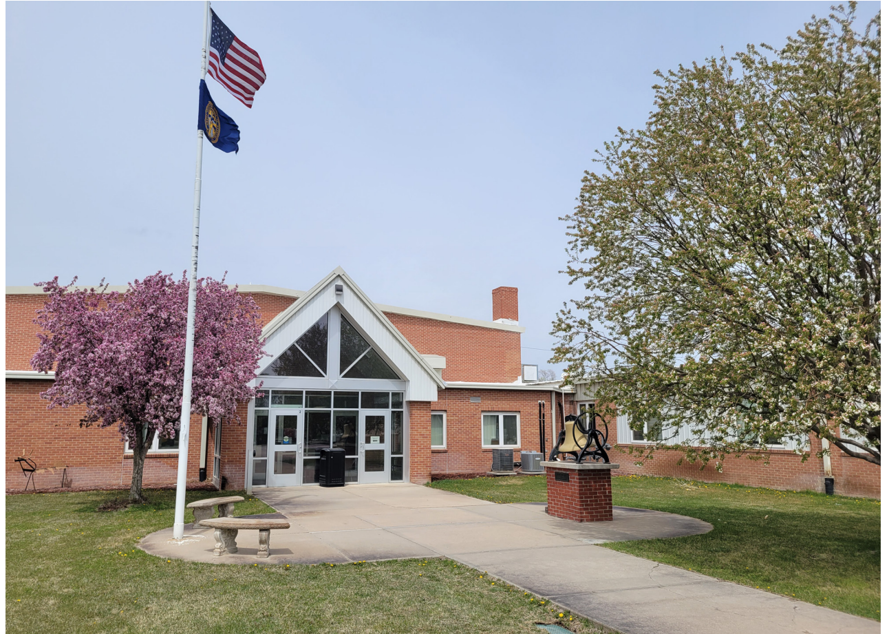
Fig. 3.4.10: School Entry Exterior, 2023.
