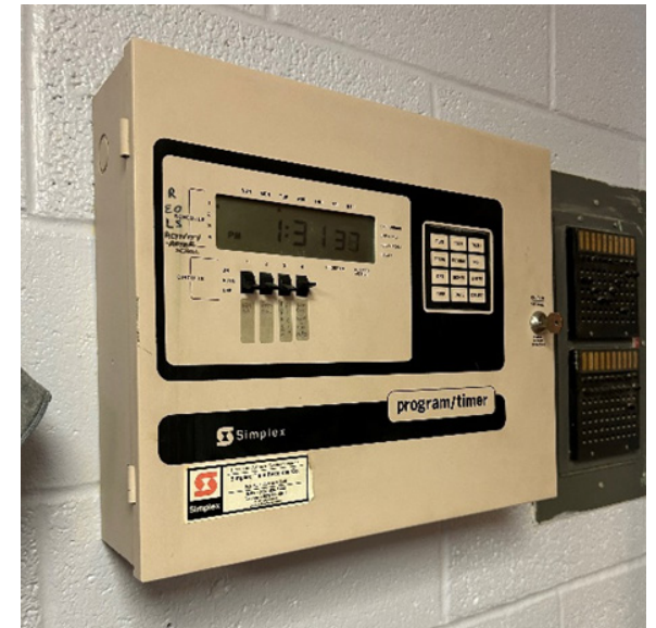
Fig. 3.6.11: Main Clock System, 2023.
