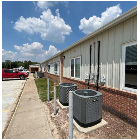
Fig. 3.5.18: Typical Split System Outdoor Air Source Heat Pumps, 2023.
